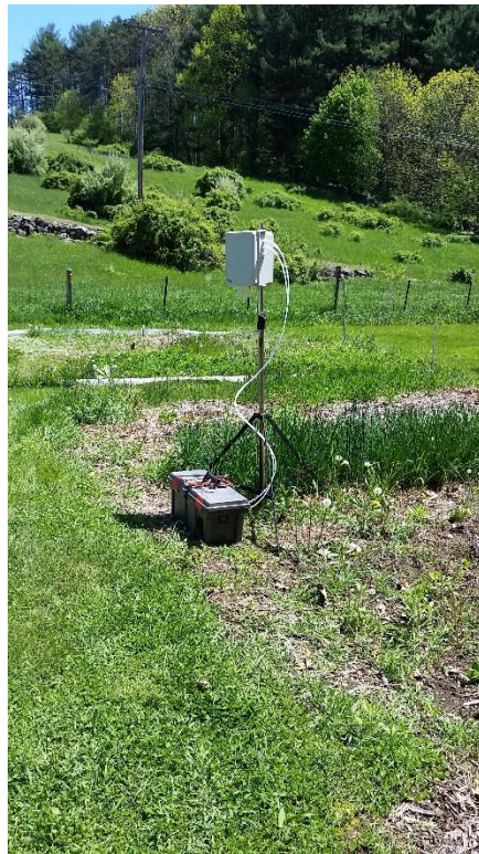
Figure 4. One of the pump monitors used at the SVSF.
